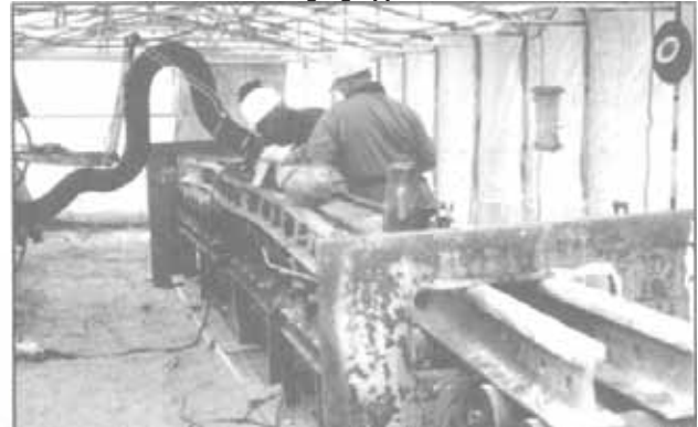
Welding Jig Application
